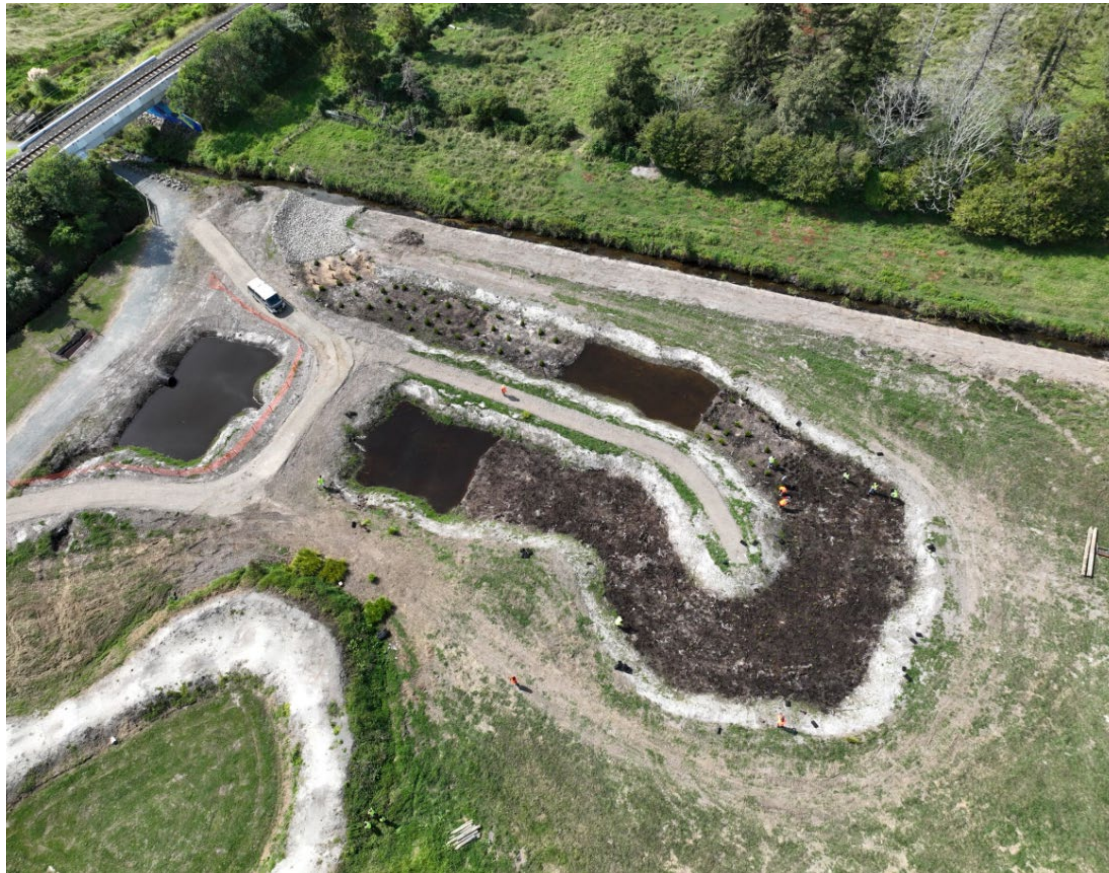
Lawrence Oliver Park wetland in Te Puke following earthworks completion (March 2025)
