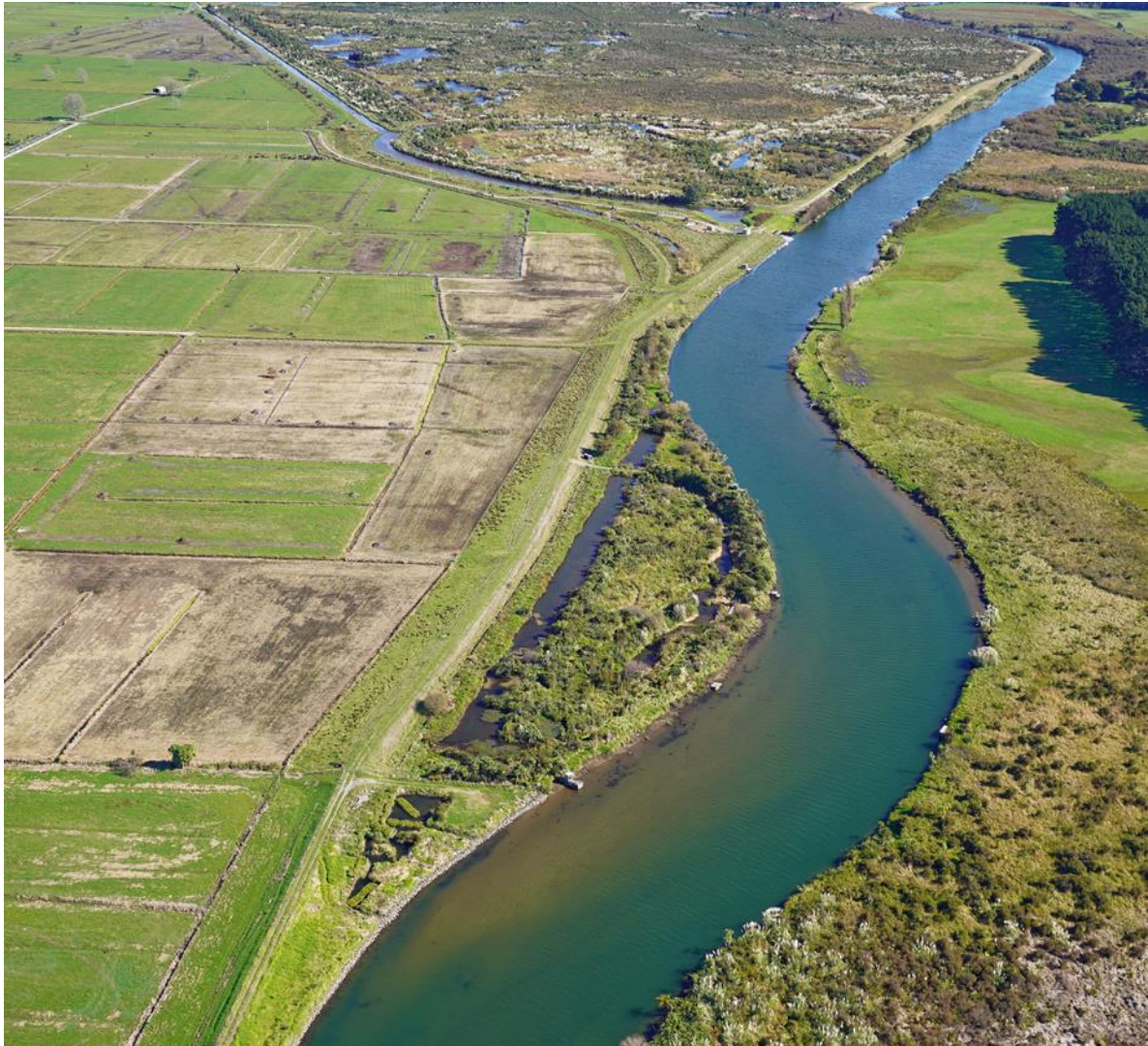
Photoblique image of Te Huauri o Te Kawa (looking upstream) with Kaituna wetland in the distance.
