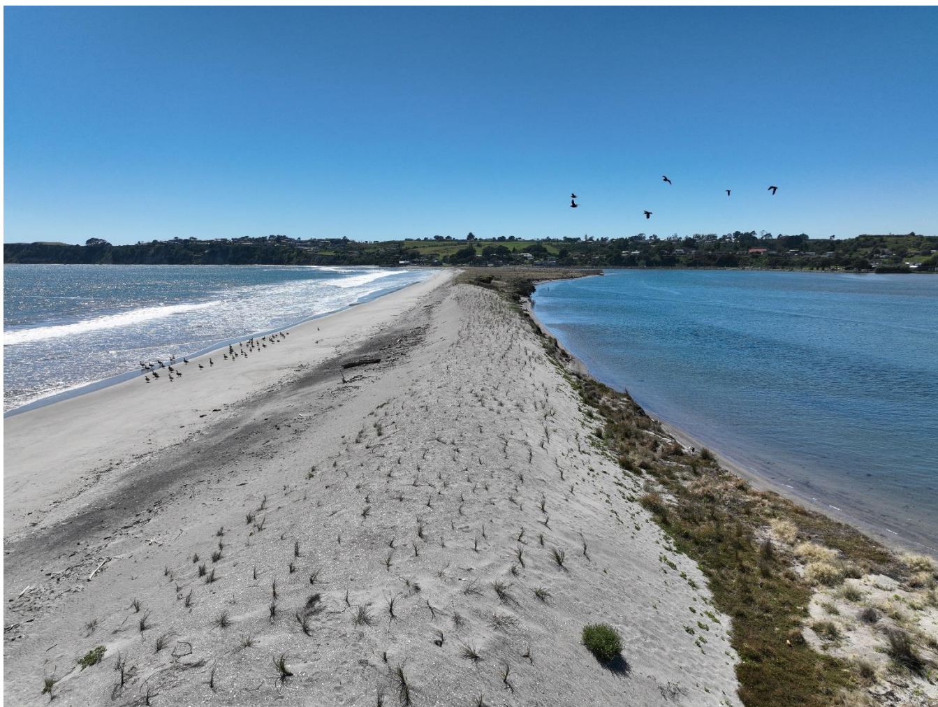
Photo showing the completed dune nourishment following planting, taken 14 th January 2025.
