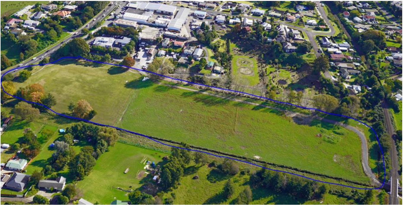
Lawrence Oliver Park in Te Puke- the future location of a constructed wetland and biodiversity area alongside the Te Ara Kahikatea walkway.
